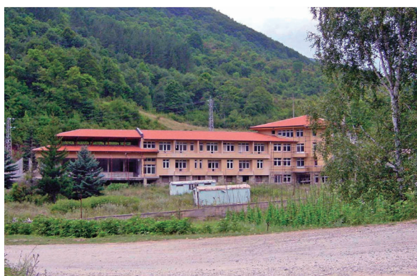
Photo 13. A new hotel under construction (8. 2005)
