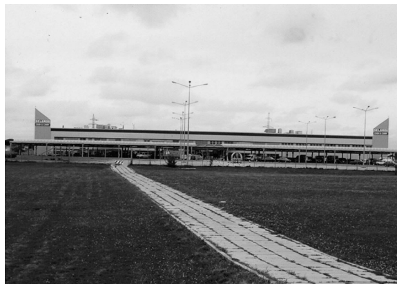
Photo 1. Pantelimon commune: new supermarket (August 2005)
